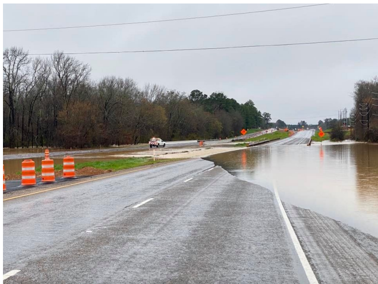
Fig. 2: Flooding on US Highway 69 near Tyler, TX on February 12, 2020 Image Courtesy of Doc Deason
